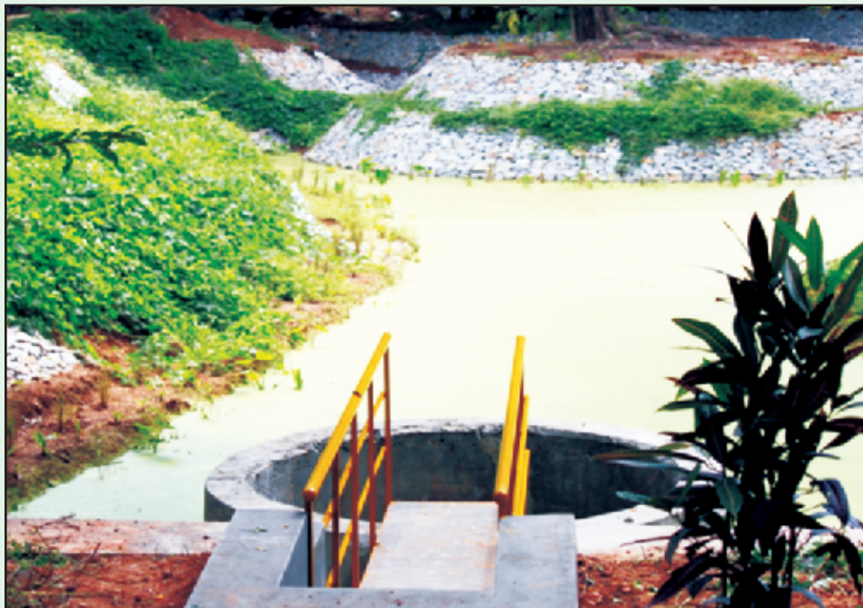
(1) Rain water harvesting system at Mysore Zoo
